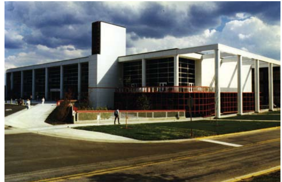
Student Resource Center addition
