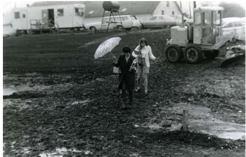
Students walking through the mud on West Campus during construction
